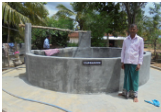
Figure 9: Agrowell constructed through project funds installed in Medirigiriya
