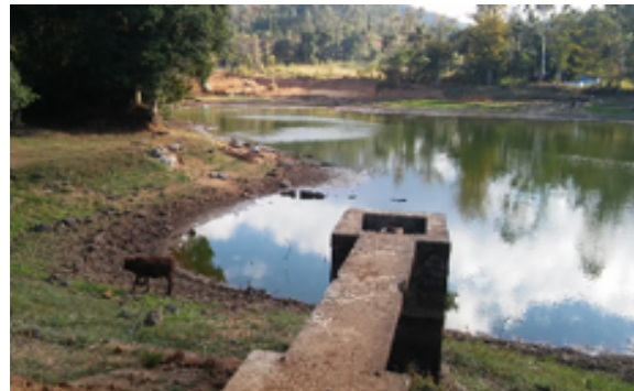
Figure 16: Minor tank rehabilitated in Walapane
