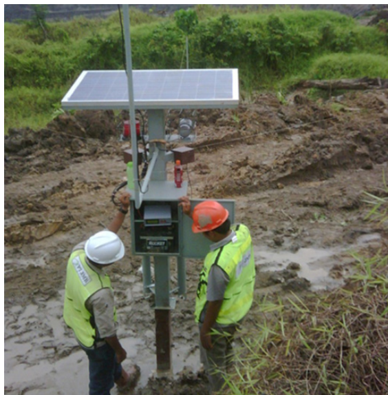
Figure 7: EW system being installed by NBRO
