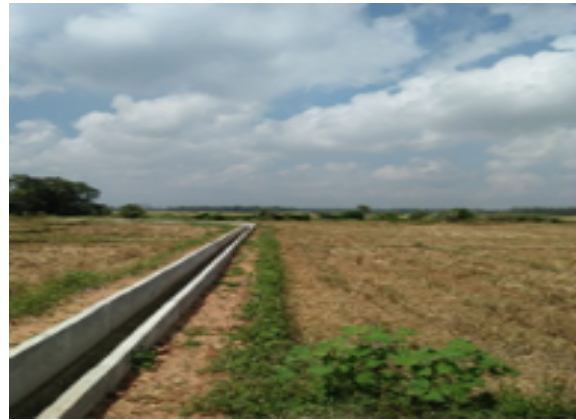
Figure 15: Canal constructed by the project in Medirigiriya
